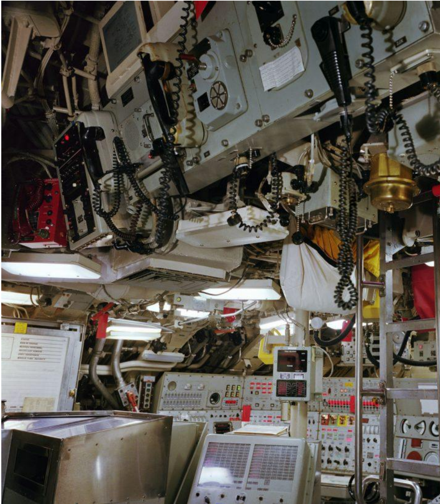
Trident submarine control room (also known as the Attack Center), USS Alaska, Naval Submarine Base Bangor, Washington. This area contains the boat's two periscopes, the Control Station from which the planesmen adjust the submarines motion, and various communication, sonar, navigation and weapons control systems. Some of the instruments seen in this photo have Velcro-mounted leather covers to conceal the classified range of depth and speed on the dials from visitors without security clearance. Paul Shambroom, 1992.
